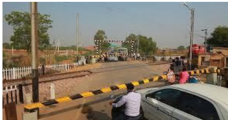
Figure 3. Modern Technology for Level Crossing [9]
