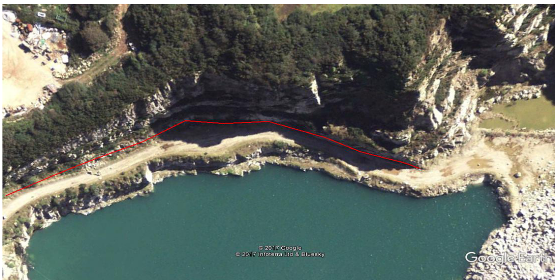
Figure 2. Section of Carnsew quarry slope on which point cloud data [1].
