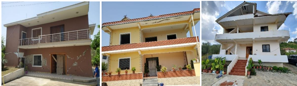
Figure 1. Building façade photos URM (left), CM (mid) and RC (right)
