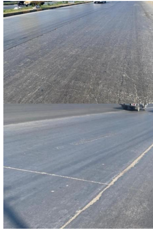
Figure 5. A field photograph of Airport Street taken by the author
