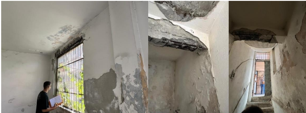
Figure 2. Building 7 Degradation and severe damage on structural walls and beams
