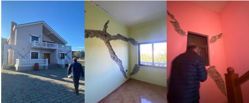
Figure 3. Building 5 Shear cracks and severe damage on URM walls
