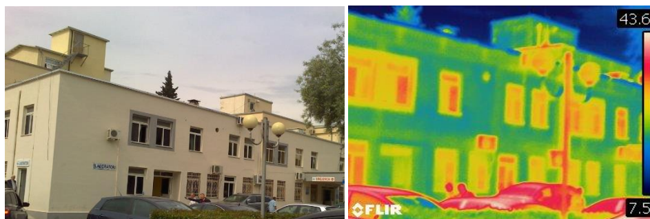
Figure 6. Image of façades from thermal camera
